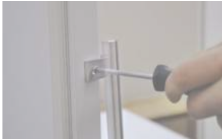
Mount the handle onto the door.
