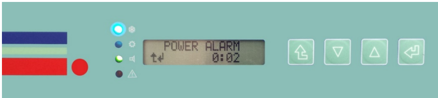
Example Power Alarm display, with 2 minutes power loss duration
